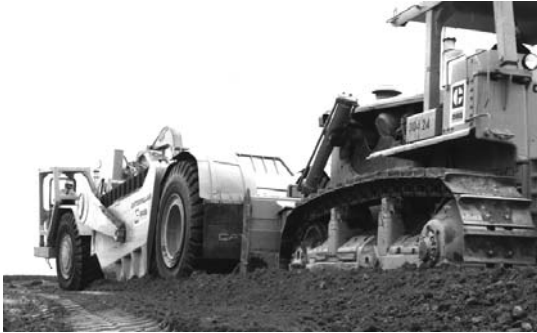
Fig. 13.12 Tractor pushing a scraper. (Caterpillar Tractor Co.)
