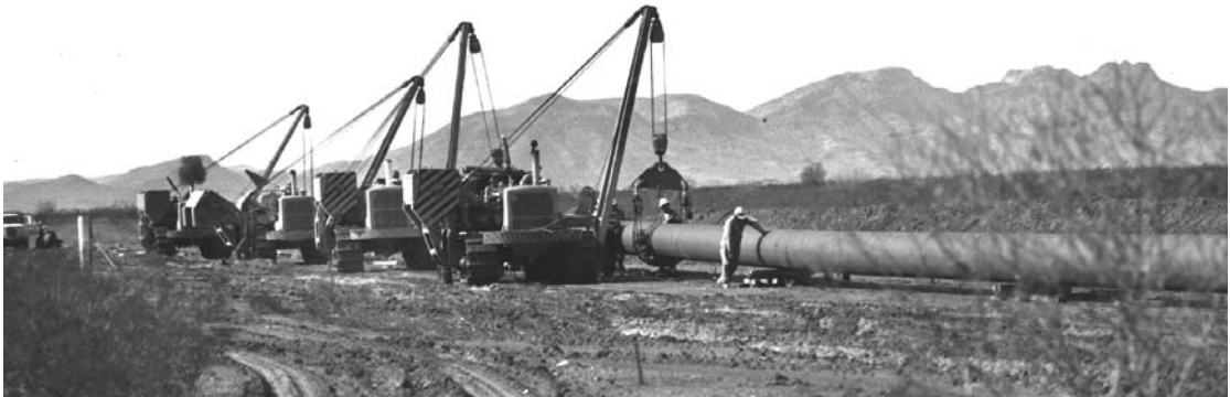
Fig. 13.11 Pipelayers. ( Caterpillar Tractor Co. )
